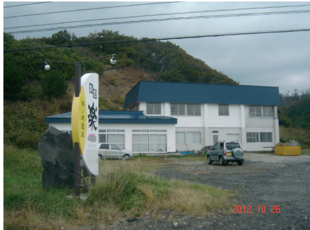
Picture 2: New processing plant under construction in October 2012
